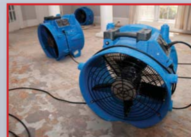
Check ambient temperature and humidity during restoration drying
