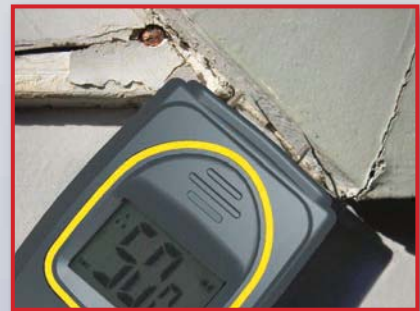
Check drywall for moisture
