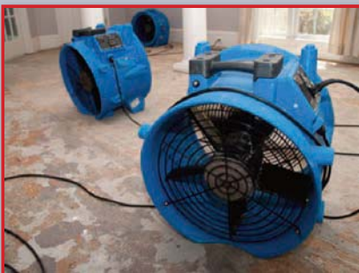
Check humidity and ambient temperature during restoration drying
