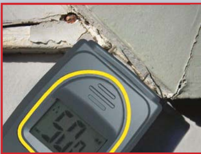
Check drywall for moisture
