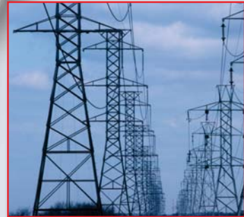
Power Distribution and Generation Maintenance
