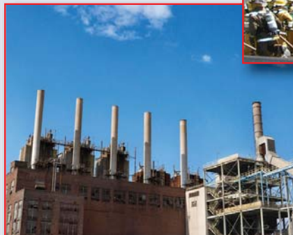
Industrial Site Inspection
