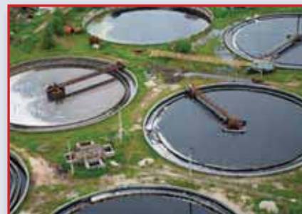
Water Pollution Control
