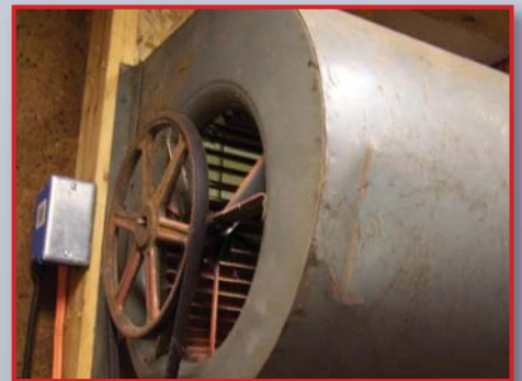
A low-speed squirrel cage blower motor
