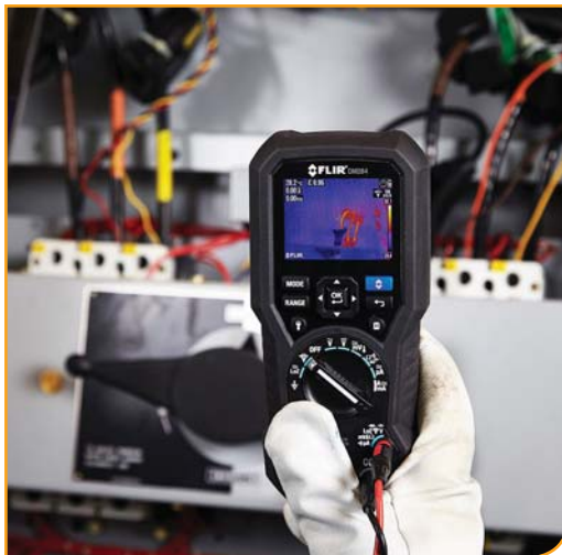
Thermal scan of an electrical panel
