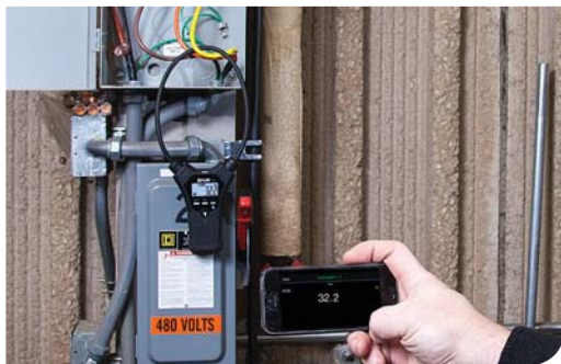
Bluetooth capability gives readings at safe distances
