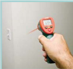
Check building for insufficient insulation
